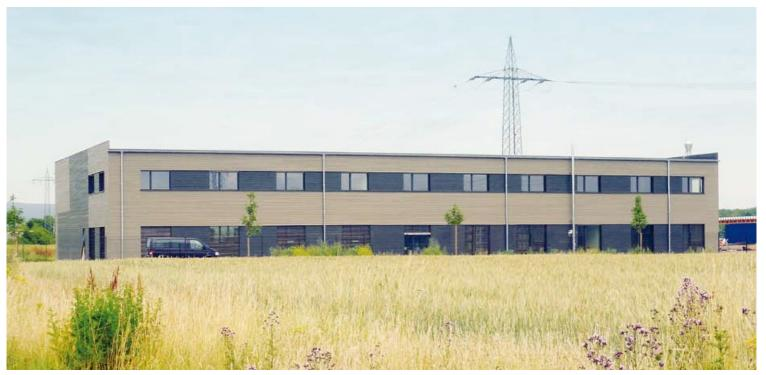
U value of the construction element from 0.088  $W/(m^2K)$  to 0.138  $W/(m^2K)$ . Even this value easily achieves the Passive House standard.
