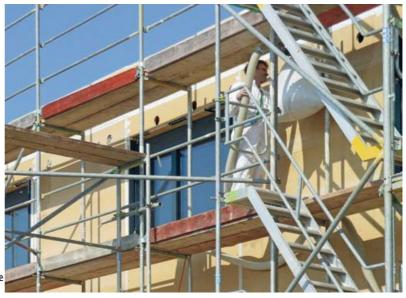
The 32 cm deep cellulose insulation is blown into the building from outside
