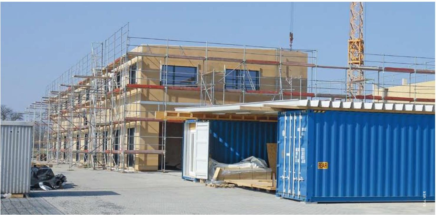
the woodworking unit had to have adequate temporary storage space. The total time spent loading is another cost factor that can be avoided.
