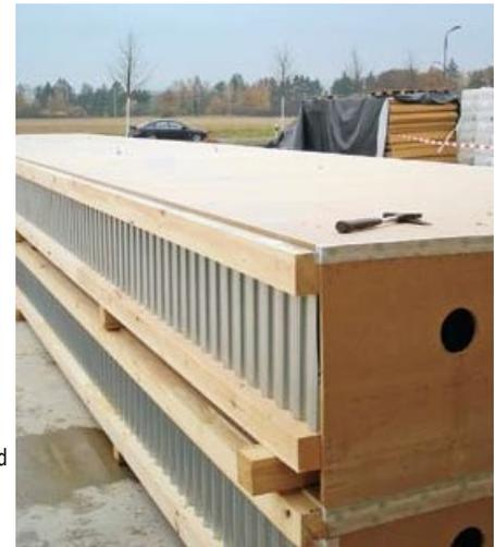
▶ The hall width of 14.50 m required 55 cm deep metal beams
