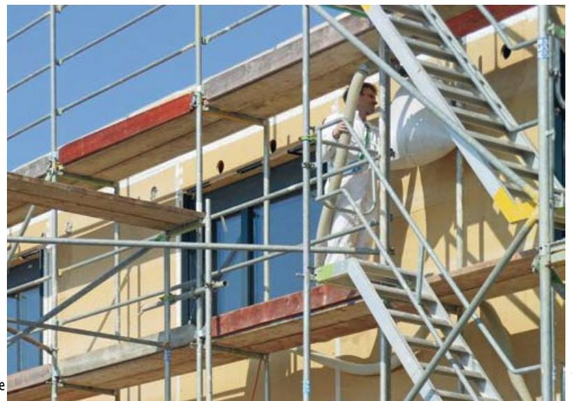
► The 32 cm deep cellulose insulation is blown into the building from outside
