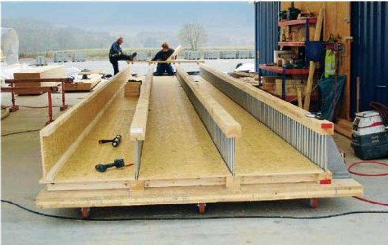
◀ Base planking was assembled from above, avoiding the need to turn the construction elements
