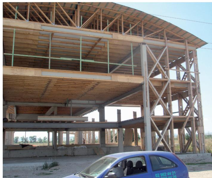
Wood is perfectly suited to transmit tensile and compressive stress in the fiber direction. Top and bottom belts in the HTS Hybridbeams bear these forces. The shear flow between the belts is provided by one or two parallel steel bars! . Thus, these beams that have been designed out of solid wood have, compared to the double beams double-T beams, an improved stability and are largely undistorted.
